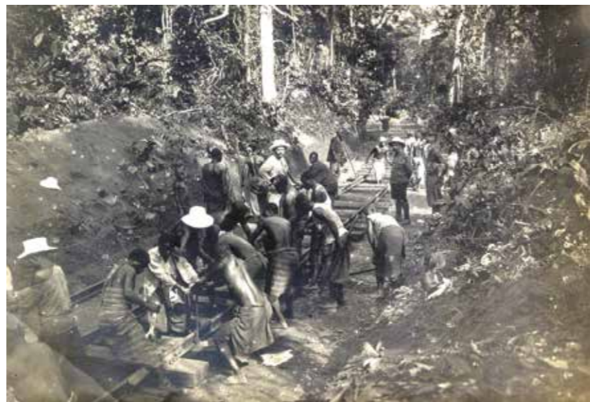
Congolese natives laying rails on the line of the Great Lakes Railway
